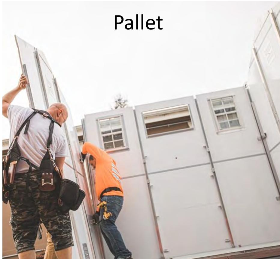
Aluminum frame, fiberglass-coated composite walls, minimal insulation / high winter heating costs, four small windows, can be disassembled for storage
