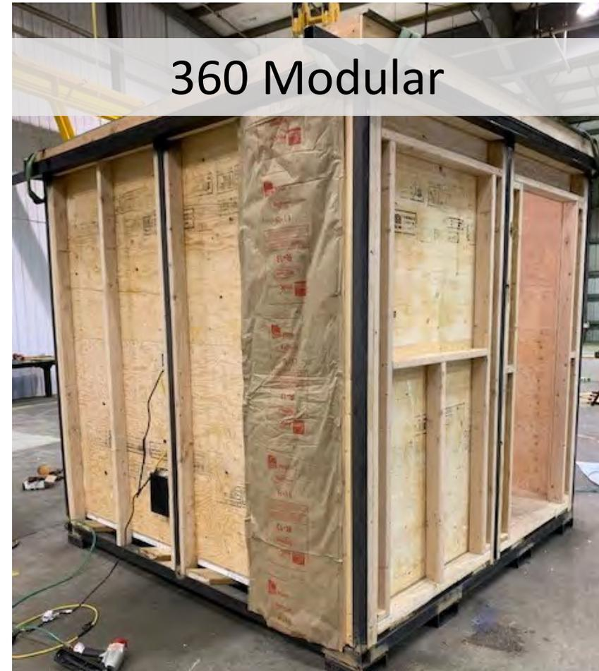
Steel structure, wood frame, R13/R19 insulation / significantly lower heating costs, one 3'x3' window, LP siding, fixed structure, "forklift and crane ready"
