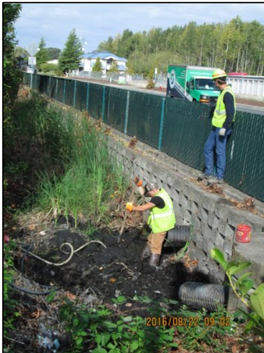
Airport Way/ Bennett Drive retention/ detention pond maintenance
