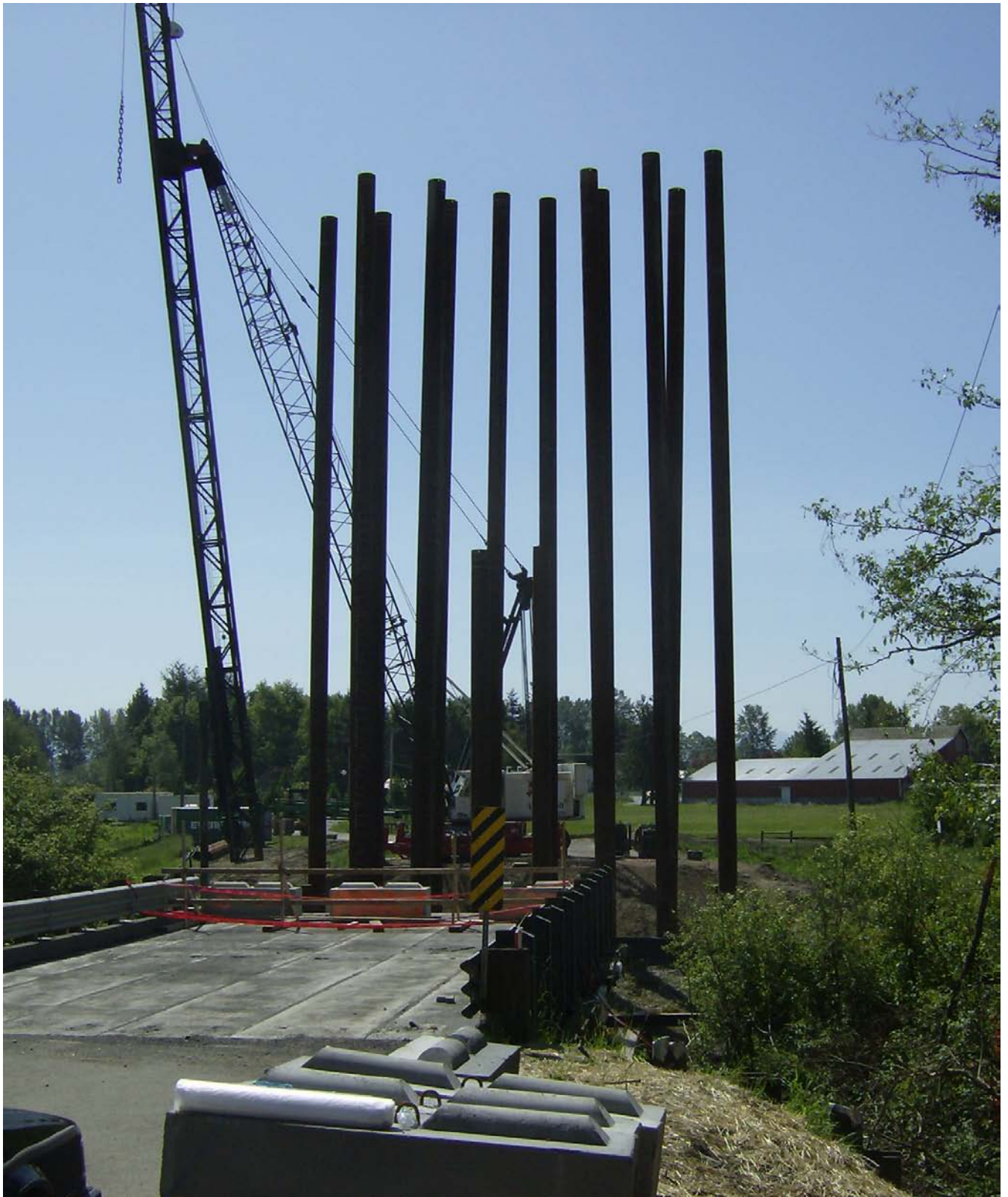
Driving the 120 ft deep pile foundation for bridge abutments
