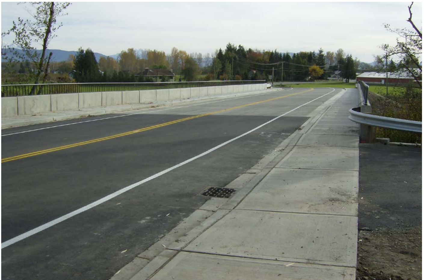
New bridge from Lynden city limits, looking south
