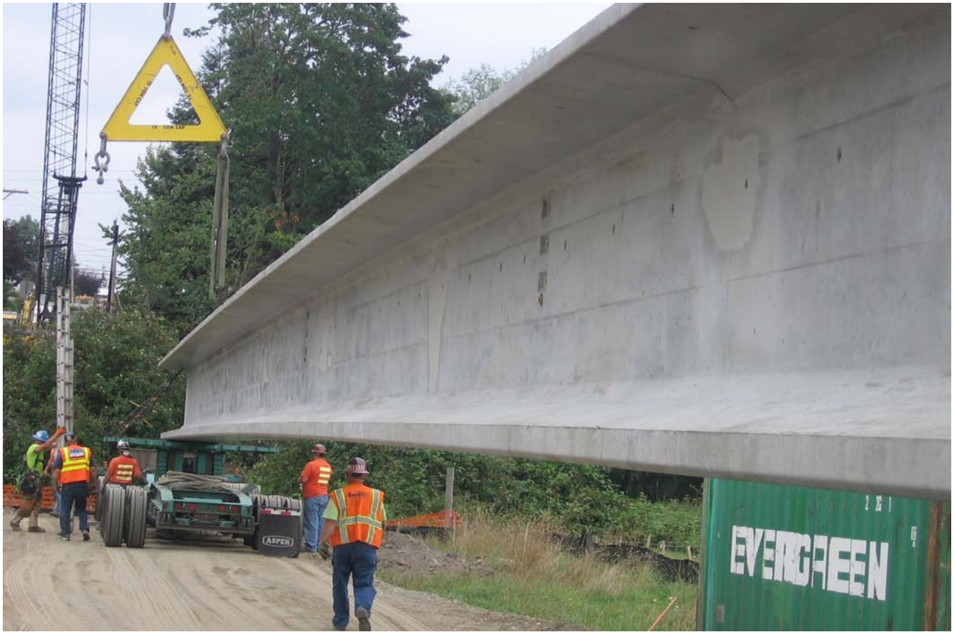
145-ft girder ready to be set
