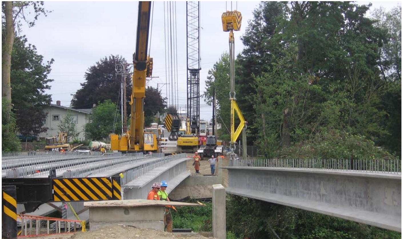
Installation of the final girder (8 total)
