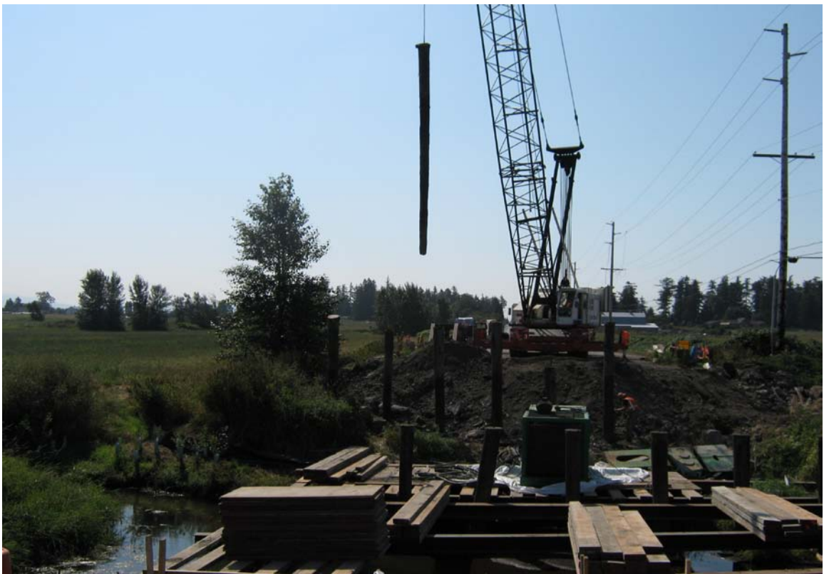
Removal of the old timber piles
