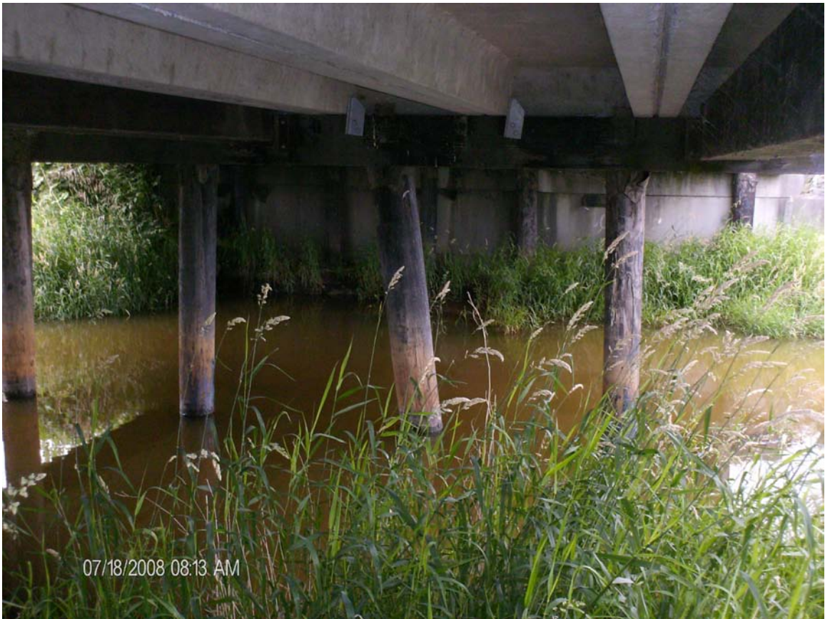
Looking north under the old bridge
