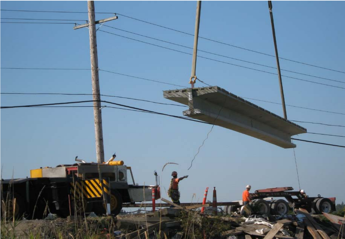
New bridge girder being set by a crane
