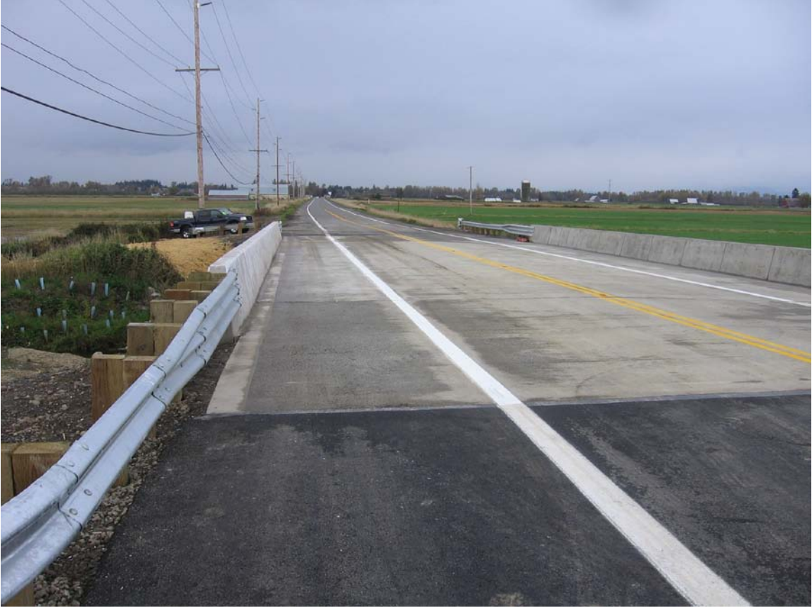
Looking north across the completed bridge
