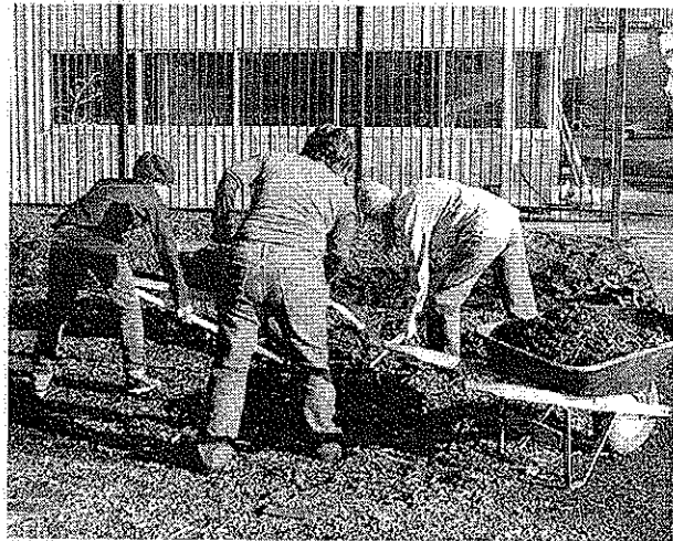
The Georgetown Community Council, working with the nonprofit Duwamish River Cleanup Coalition, helped lead the construction of stormwater swales.
