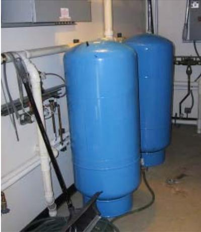
Chapter 5 explains how to make well pumps and pressure tanks work together as a single system capable of reliably providing safe drinking water to customers of new Group B water systems.
